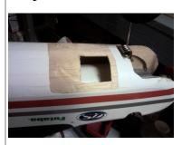
I started by clean up the damage area. I removed some covering to make clean edges and then cut the hole into a rectangular shape for easy patch.
